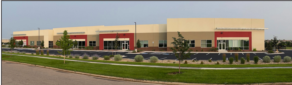
The 40,000-square-foot Racine Industrial Park, located at 6281 S. Racine St., includes four units and a secured, fenced yard.
